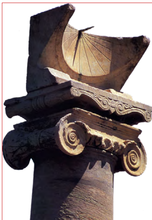
Roman hemicyclum sundial reading unequal hours (12 hours from sunrise to sunset). Thus, the daylight hours were longer in summer than in winter Such dials would typically be in a town market place.
