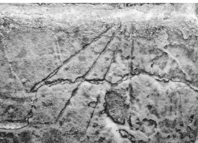
Fig. 10. Knaresborough, St John. An example of a dial with lines below the horizontal only and the gnomon hole blocked.
