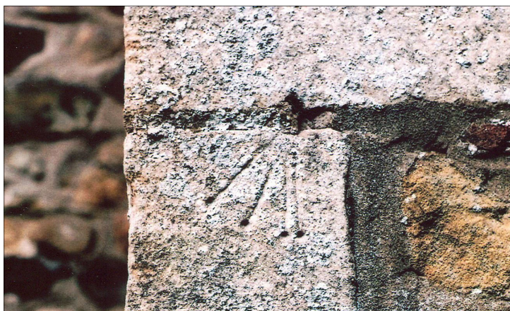
SIGGLESTHORNE, St Lawrence Church. A good example of a simple four line mass dial, type F. It has pocks at the ends of the lines and a blocked gnomon hole.
