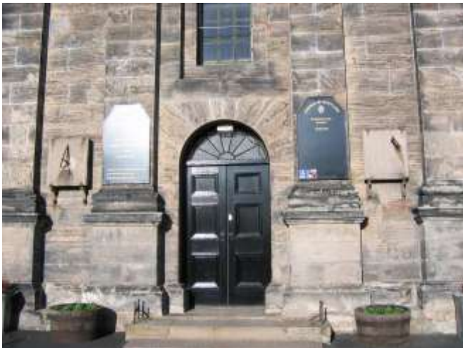
Fig. 10. The main entrance of Inveresk church showing the two dials.
