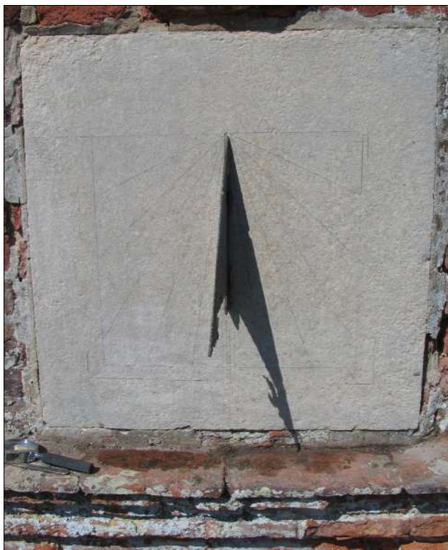
Fig. 5. After cleaning. The border and hour lines are enhanced with pencil.
