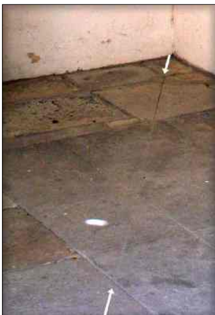
Fig. 5. The best preserved part of the line with the elongated spot of sunlight, photographed at local solar noon, showing the large error in time (Photo credit Lindsey Kerr, NPIA).
