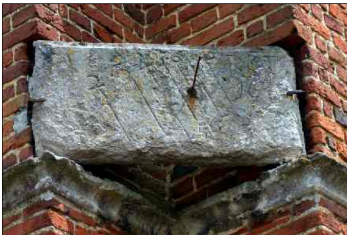
Fig 11. A close up of the vertical dial with the rusted horizontal rod gnomon.
